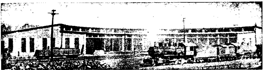
Casa de Máquinas del Eign Joliet and Eastern Railroad. Vista general.
